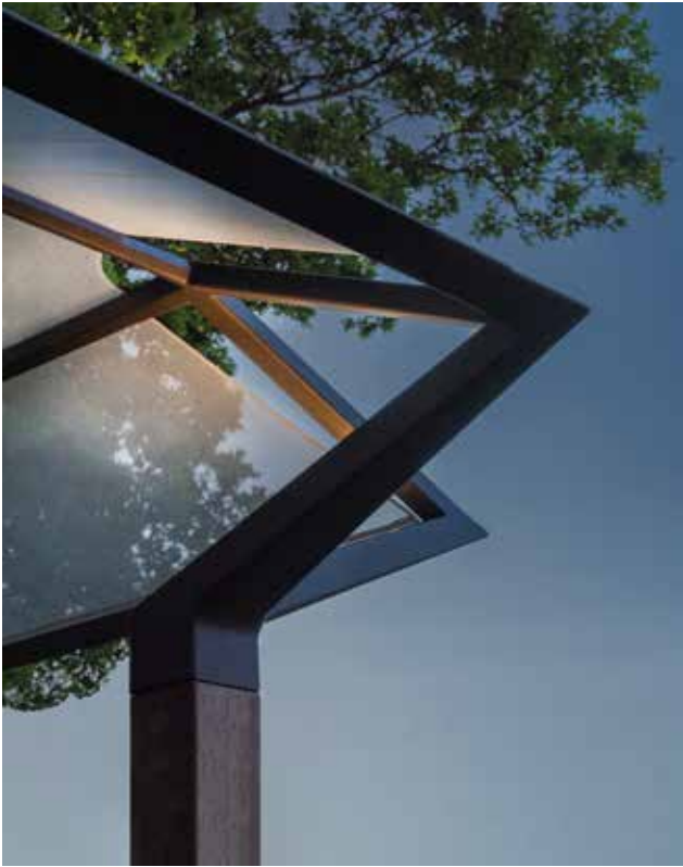
Pavilion with brushed teak columns and aluminium frame. Micro-perforated waterproof shading cover.
